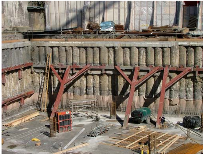
Figure 4 Secant Pile Wall, Dunnes Stores, Georges St., Dublin (Murphy International Ltd)
