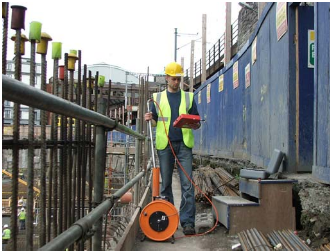
Figure 12 Inclinometer instrument being lowered into position
