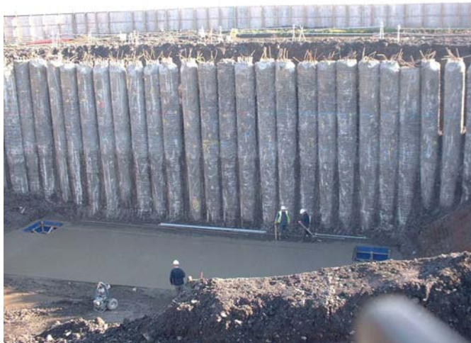
Figure 3 Contiguous Pile Wall, Dublin Port Tunnel (PJ Edwards & Co.)
