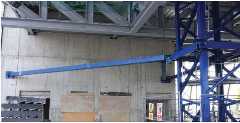
11 The South West r.c. core, with temporary crane 'tie-backs' attached – May 2008
